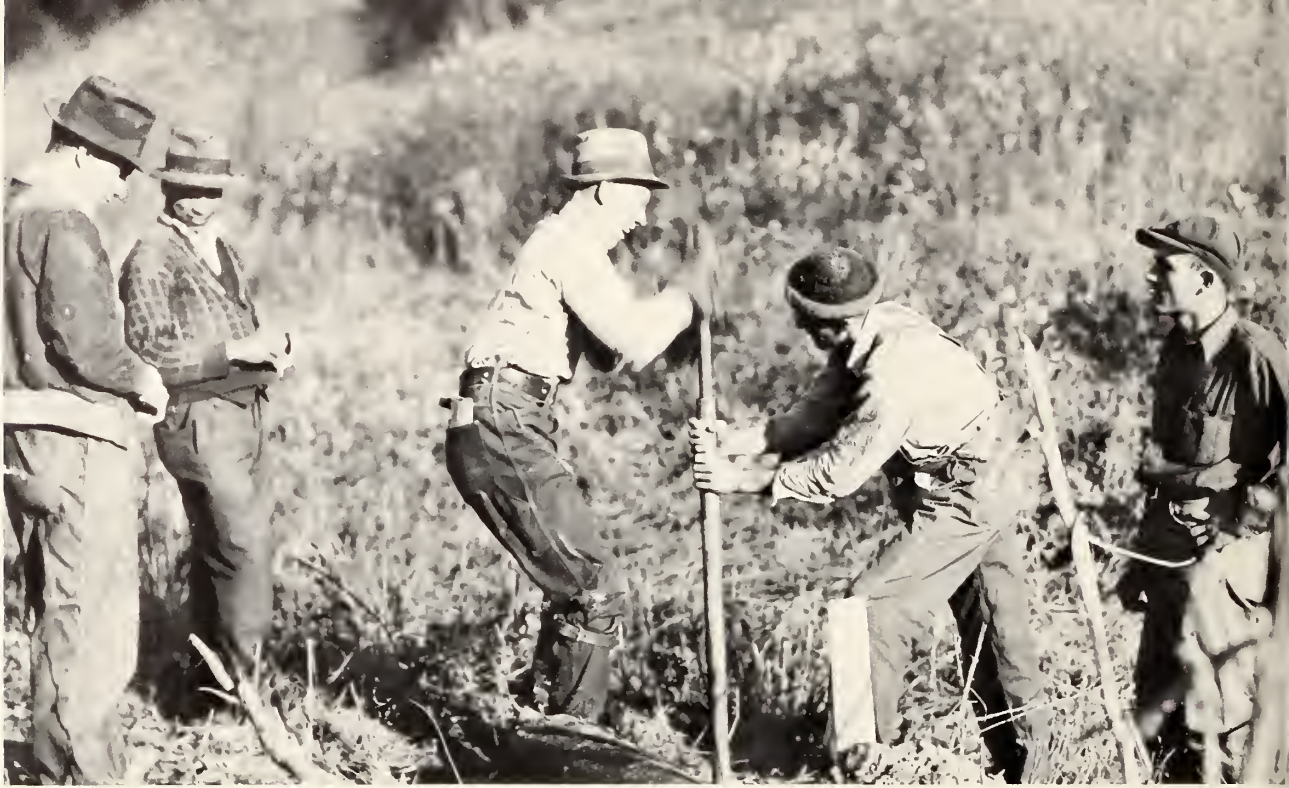
Early crews had few power tools to work with. Holes were dug by hand . . .
